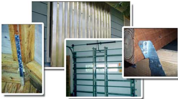
Examples of roof strapping, storm shutters and a wind-resistant garage door. Geraldine Schaeffer had all three installed on her Escambia County home.
